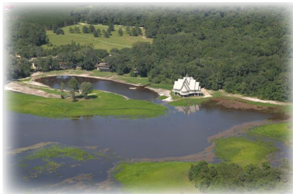
Aerial view of Episcopal Retreat Center
